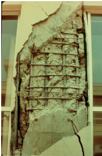
Damage class IV: Exposed rebars without buckling or fracture
