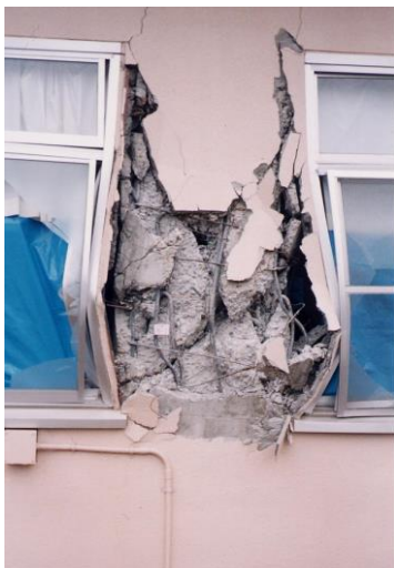
Damage class V:
