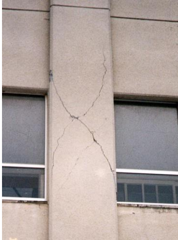
Damage class III: (left) Cracks with a width of about 2mm on structural concrete (right) Spalling concrete cover and slightly exposed rebars
