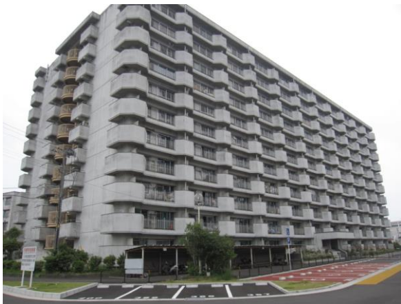
(a) Overall view
