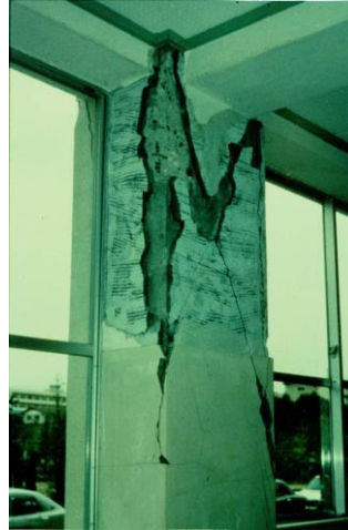
Damage class III: (left) Cracks with a width of about 2mm on structural concrete (right) Spalling concrete cover and slightly exposed rebars
