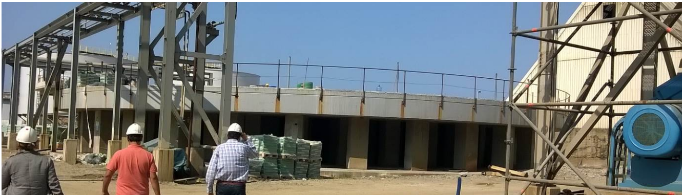
Fig. 1 – Picture from the site: existing concrete slab and foundation.
