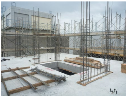
(a) Wall and column rebar
