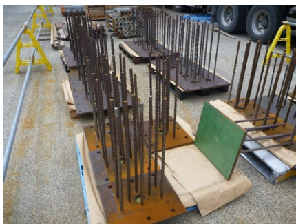
(a) Joint steel plates
