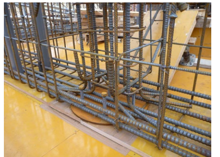
(c) Cast iron and footing beam rebar
