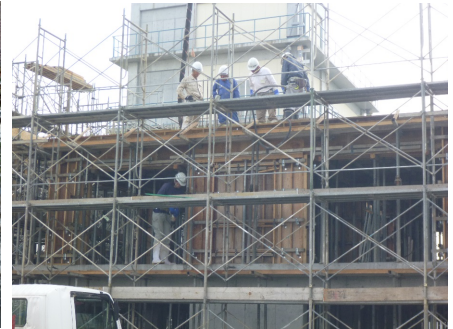
(c) Concrete placing
