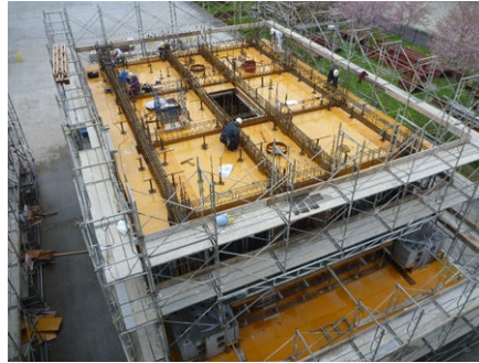
(b) Beam rebar
