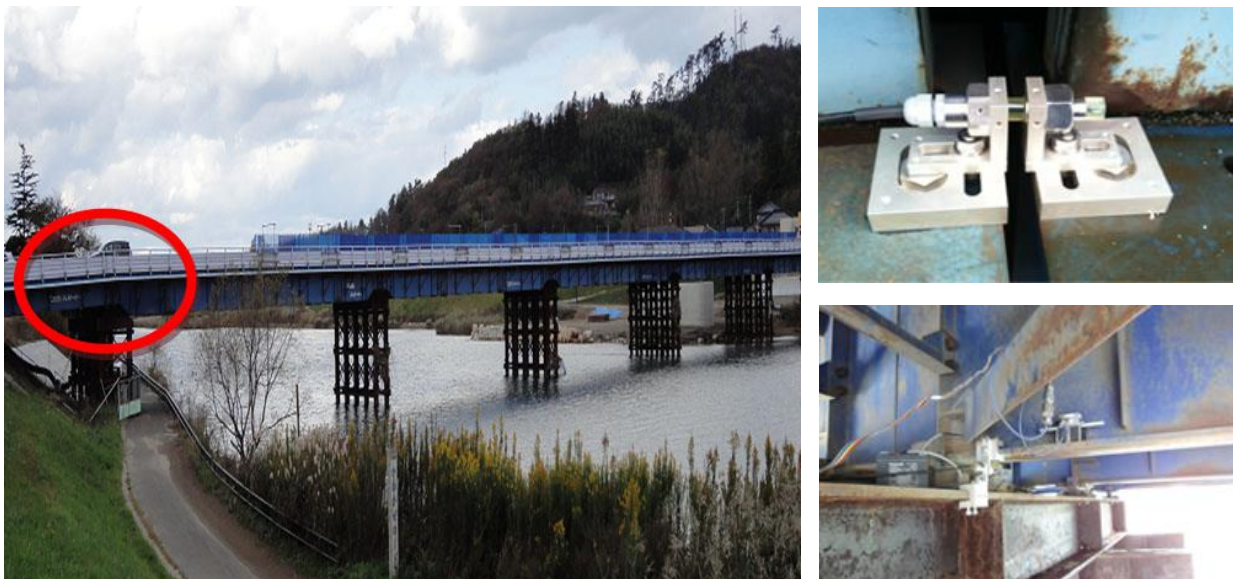
Fig. 4 – Temporary bridge for preliminary measurements
