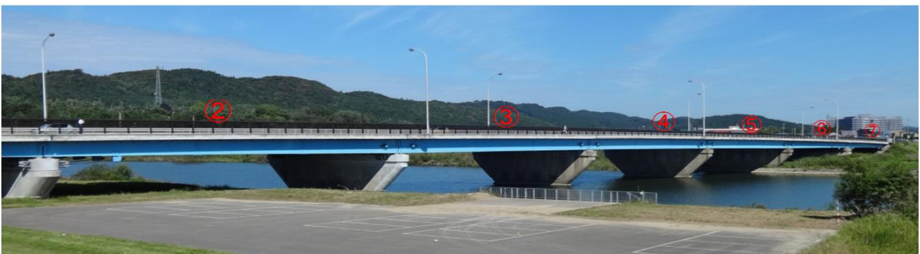
Fig. 6 – Asuka bridge chosen for measurements with piezoelectric sensors
