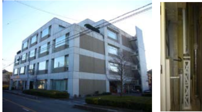
Fig 13 -A mid-rise building to which this system was introduced
