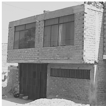
Fig. 1 – Typical CM building
