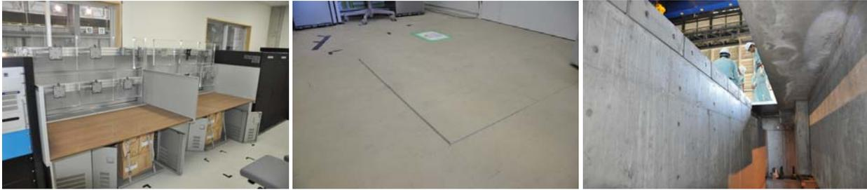
Photo 2 Damage after Pounding to BW20 under Tennoji 72% Excitation (Case 3)
