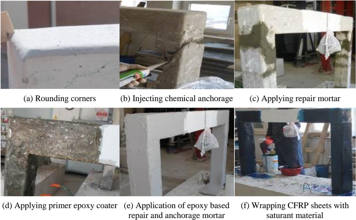
Fig. 2 - Repairing procedure for the damaged captive columns
