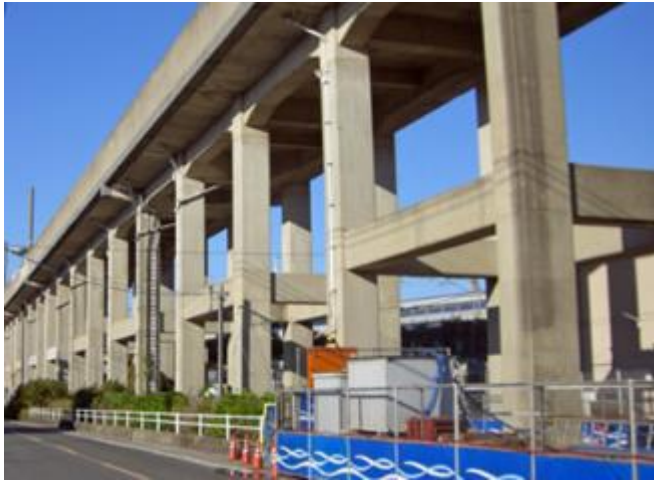
Fig. 1 – Rigid-framed railway bridges
