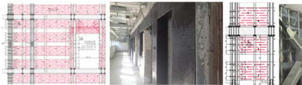
Fig. 13 - FRP and steel plate concrete wall strengthening and its implementation on site
