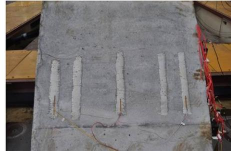
Figure 11 – Cracks in the arch springing of RC arch model
