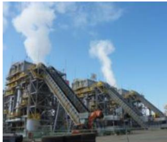
Fig.4: Debris Operation site in Ishinomaki, Miyagi [3].
