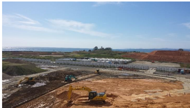
Fig. 13: Land preparation for a housing project in the Kesennuma area (Sept. 2015).
