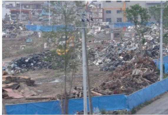
Fig. 7: Temporary storage site of debris in Ishinomaki City, Miyagi Prefecture (photo by T. Norton June 2011).
