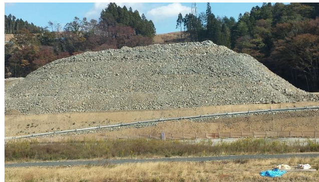
Fig. 15: Disaster waste storage piles for use in reconstruction projects (photo by T. Norton Oct. 2015).
