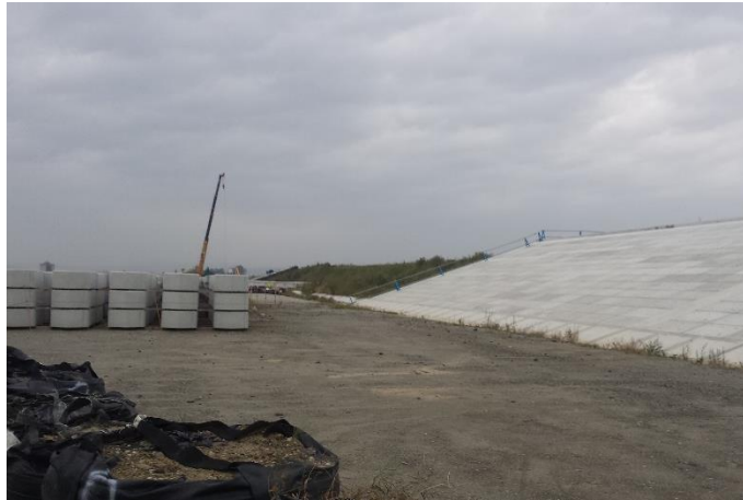
Fig. 17: Levee under construction in Natori City (photo by T. Norton Oct. 2015)
