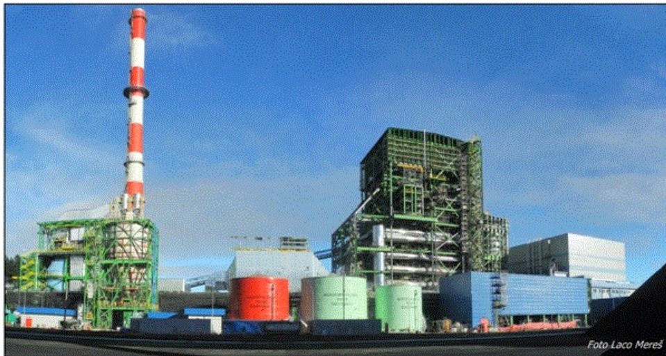
Fig. 1 – View of a Colbún power station
