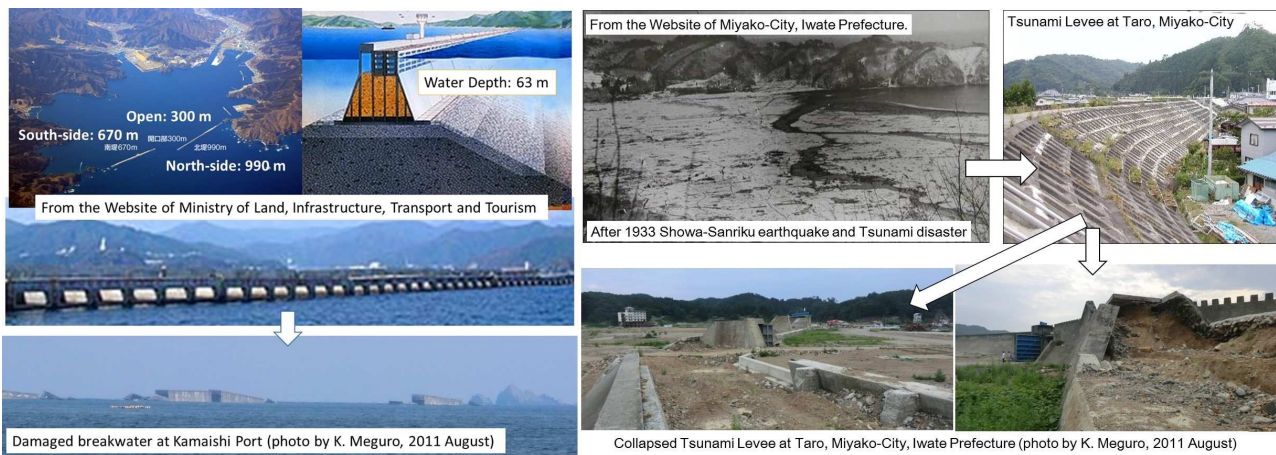
Fig. 2 – Damage to structural countermeasures against tsunami, breakwater at Kamaishi Port (left) and tsunami levee at Taro, Miyoko-City, Iwate Prefecture
