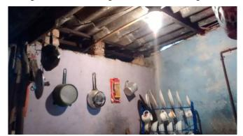
Fig. 5 – Masonry wall without top beam
