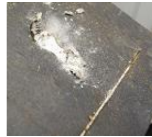
(c) Cut off of metal lath
