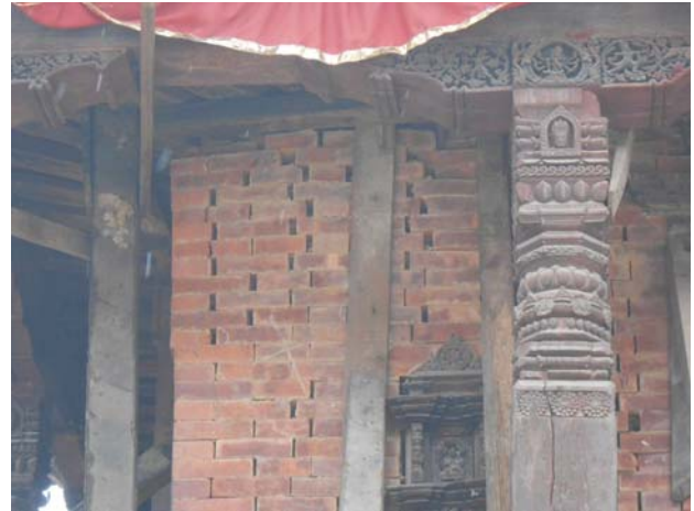
Fig. 4 – Delamination of multi-leaf wall veneer (left); diagonal sliding shear failure (right).
