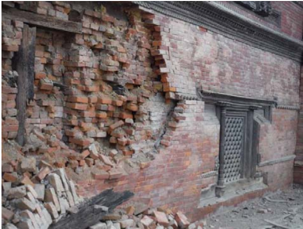
Fig. 4 – Delamination of multi-leaf wall veneer (left); diagonal sliding shear failure (right).
