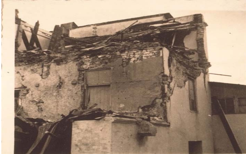
Fig. 1 – Upper part of a house that collapsed in the 1939 Accra M6.5 earthquake
