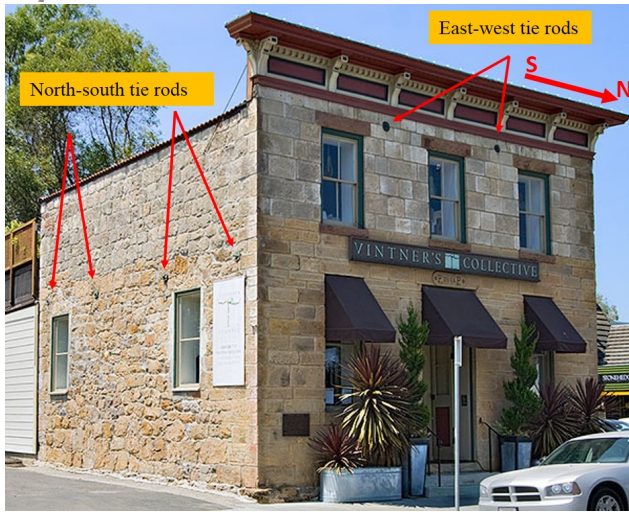
a) Reinforcement measures
