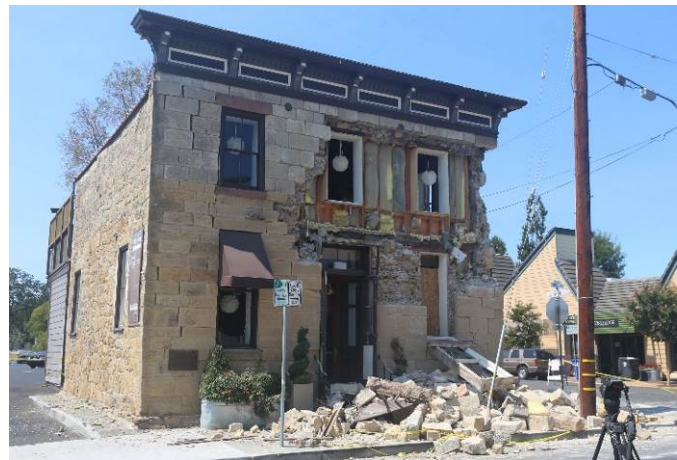
b) East and south walls
