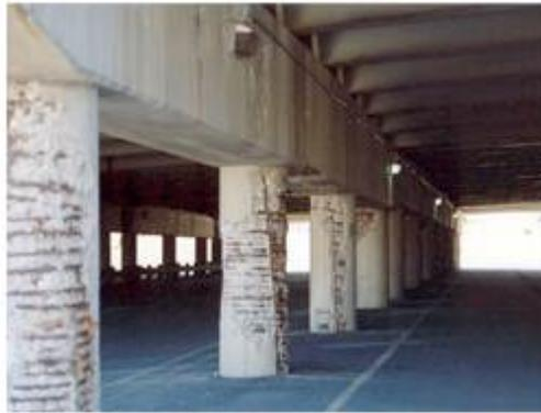
Fig. 1 - Highway bridge with corrosion damage
