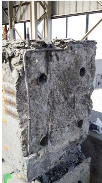
Fig. 4 – End-section of the beam, after testing
