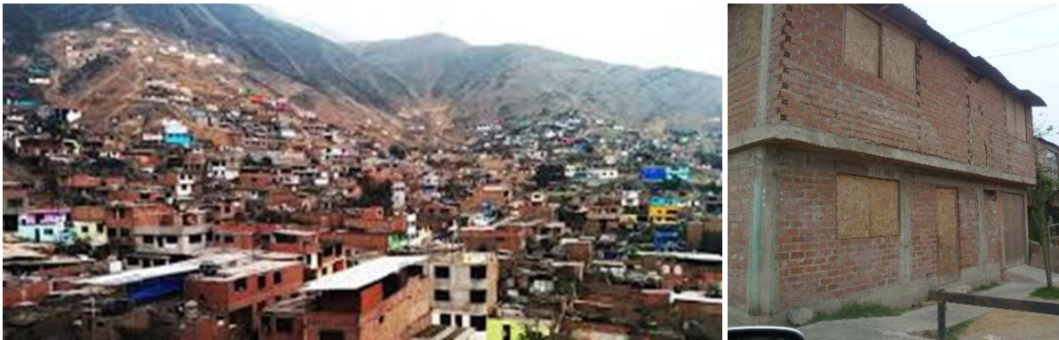
Fig. 1 – Non-engineered dwellings of masonry in emerging towns of Lima
