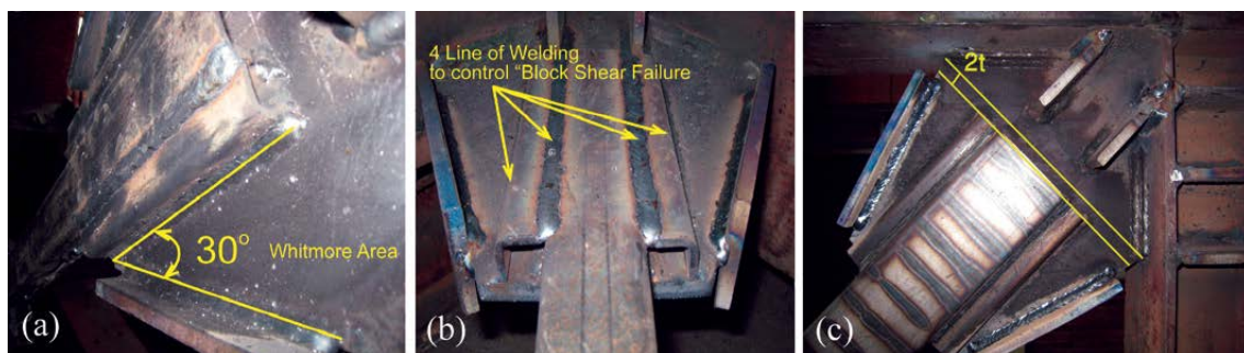
Fig. 4 – Gusset Plates Design Considerations, a) Whitmore Area, b) Block Shearing Failure, c) 2t distance at end of braces
