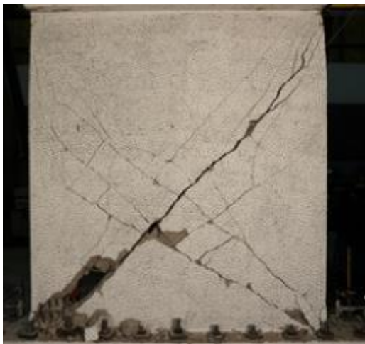
c) Ductile diagonal tension failure, WSL5
