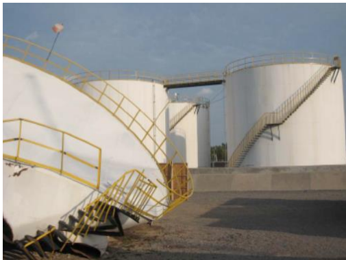
Figure 7. El Maule 2010, Chile earthquake. Collapsed water tank nearby liquid fuels tanks, Santiago Airport.
