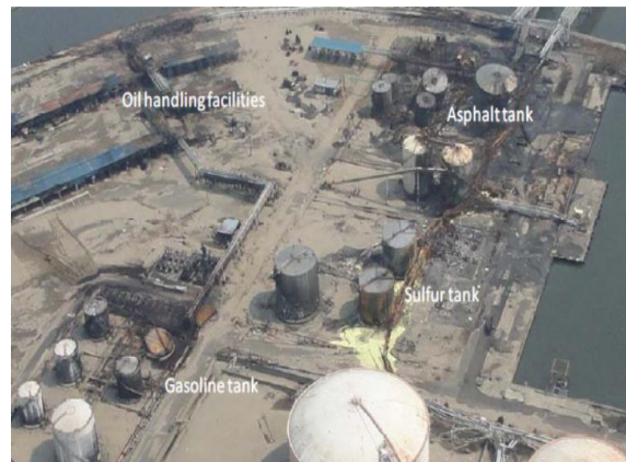
Figure 20. Burned-out zone refinery, 2011 Japan Earthquake [27].
