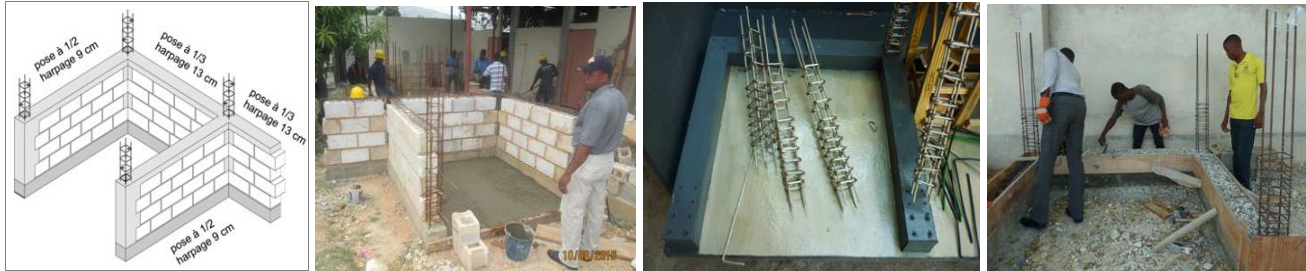
Figure 8: a) The F-structure, b) fixed vertical reinforcement with masonry and seismic bands reinforcement, c) model with holes in the plinth beam for variable wall lengths, d) re-useable material for the plinth beam.
