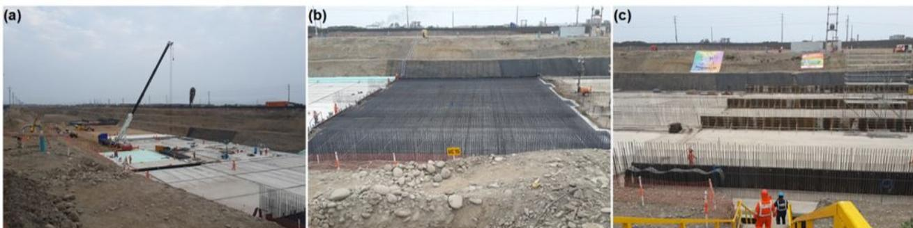
Fig. 12 – (a) Excavated trench. (b) Bottom slab reinforcing. (c) Bottom slab and wall dowels.
