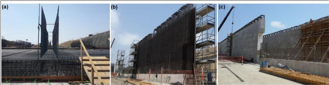
Fig. 13 – (a) Bottom slab reinforcing and wall dowels. (b) Wall reinforcing. (c) Walls.
