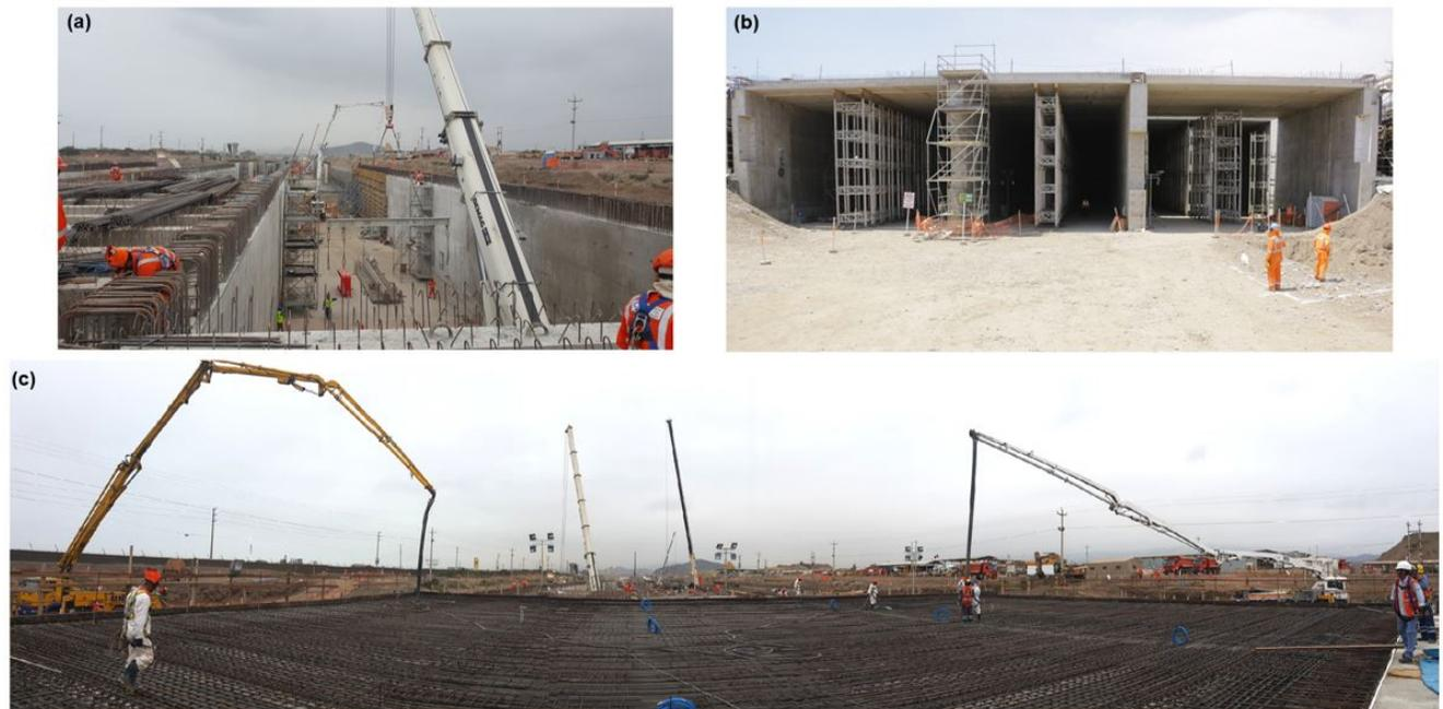
Fig. 14 – (a) Erection of precast inverted T-beams. (b) Precast inverted T-beams set on walls. (c) Roof reinforcing.
