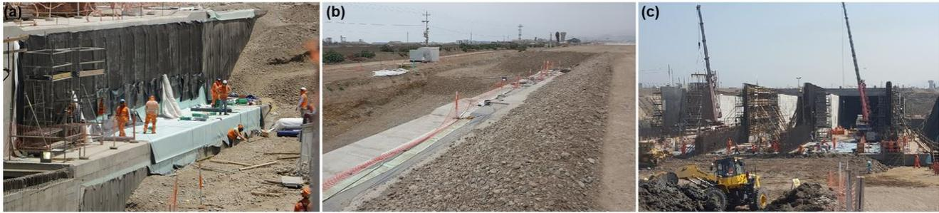
Fig. 15 – (a) External waterproofing system. (b) Fill cover over roof. (c) Open trench construction.
