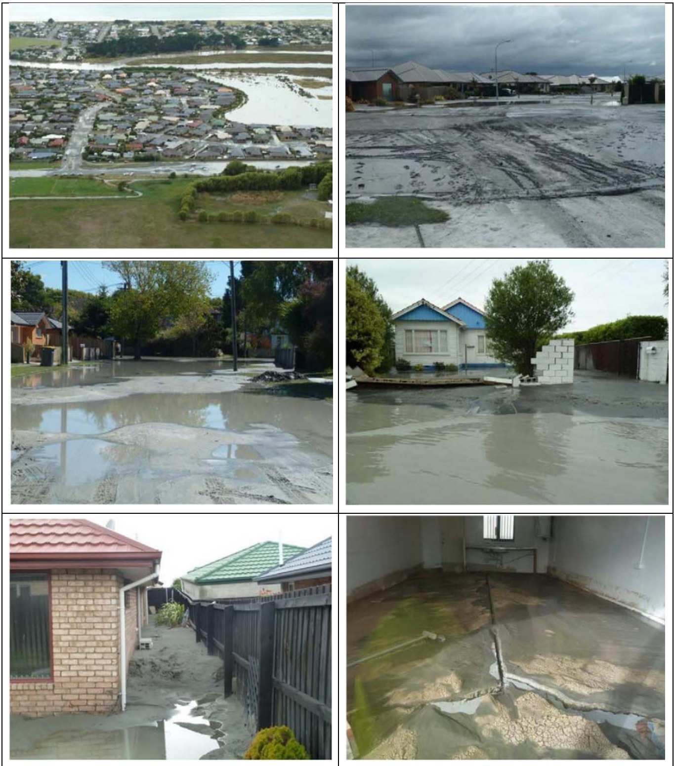
Fig. 1 Observed liquefaction related land damage and residential house damage in Christchurch following the CES [3]
