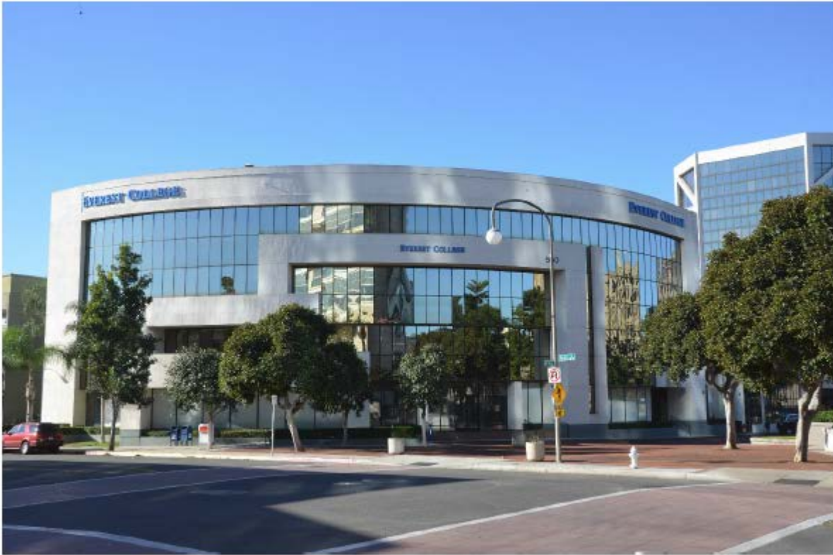
Fig. 1 – Building North and East Elevations
