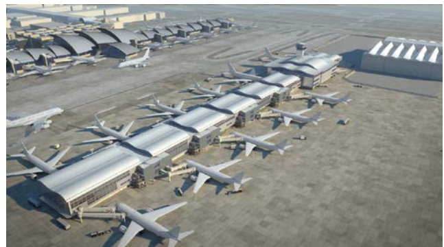
Fig. 2 – Overall View of New Terminal Building
