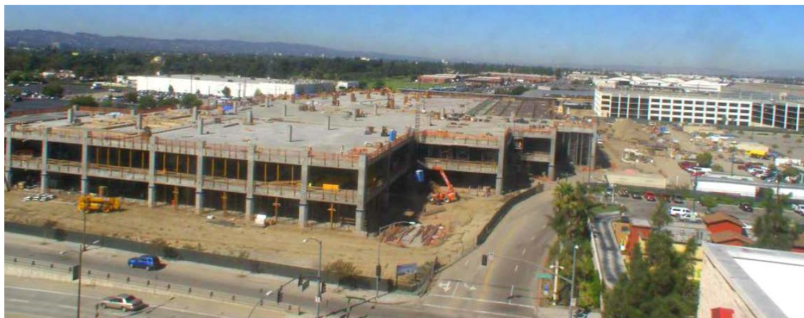
Figure 9 – Construction Photo Showing Completed Reinforced Concrete Portion of Structure
