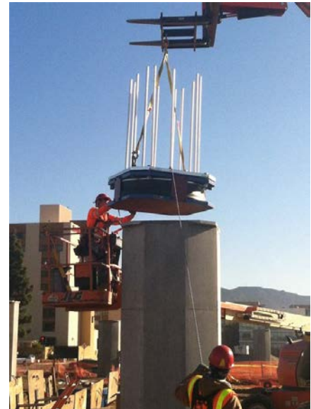
Figure 8 – Construction Photo Showing Triple Friction Pendulum Isolators
