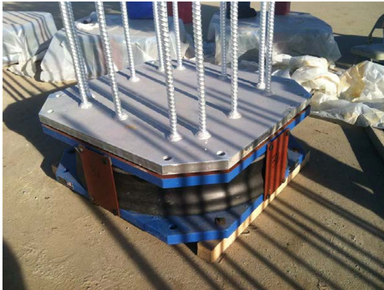
Figure 8 – Construction Photo Showing Triple Friction Pendulum Isolators
