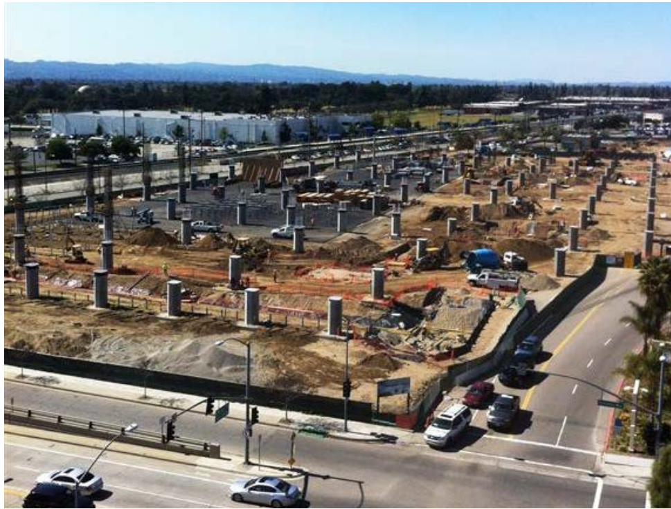
Figure 7 – Construction Photo Showing Completed Foundations and Cantilever Columns
