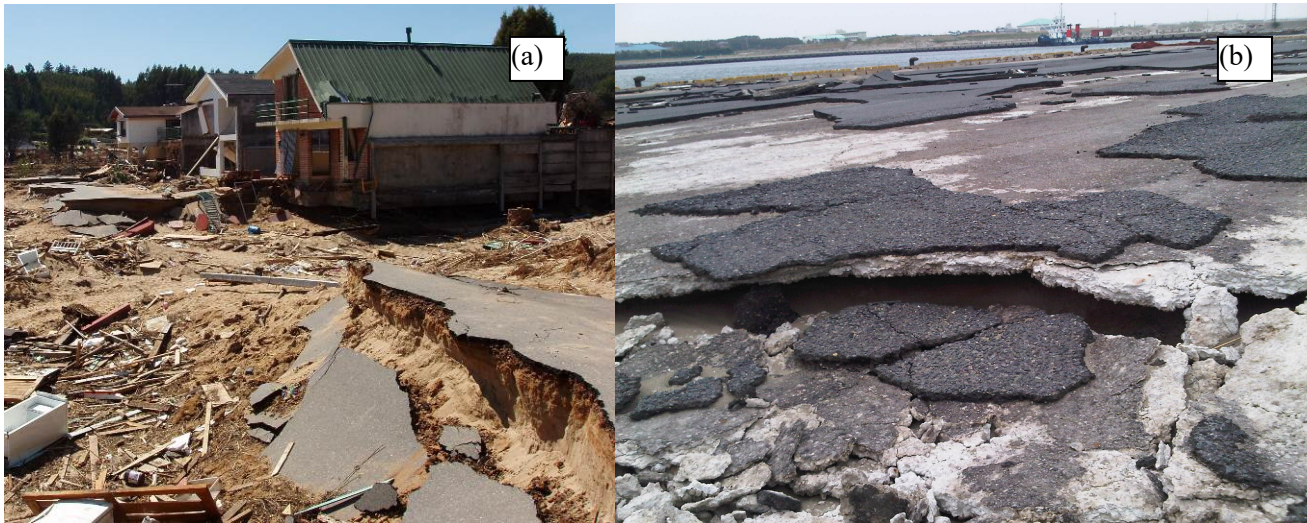
Fig. 10. (a) Roadway damage at Dichato, Chile after 2010 Maule earthquake and tsunami. (Photo courtesy C. Petroff). (b) Hasaki Port, Japan, pavement scour, Tohoku earthquake and tsunami. (Photo courtesy M. Francis).
