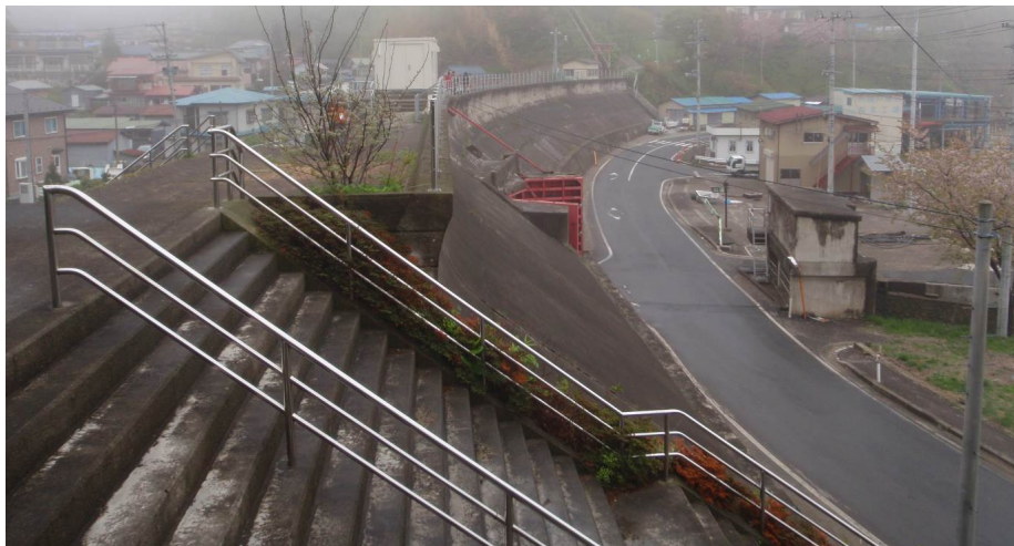
Fig. 8. Fudai Village tsunami barrier, Fudai, Japan. The houses on the left side of the photograph were completely protected by the barrier during the Tohoku tsunami event. (Photo courtesy Y. Tanaka).
