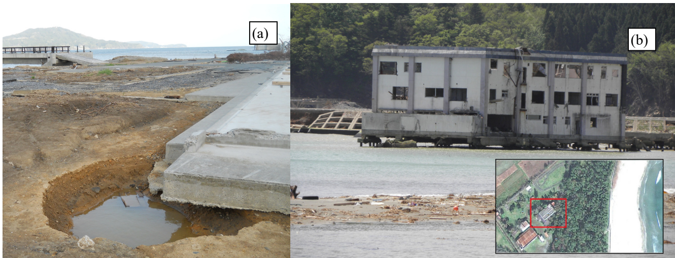
Fig. 1 (a). Local scour around building corner at Rikuzentakata after 2011 Tohoku tsunami. (Photo courtesy B. Jones). (b) General erosion in combination with subsidence of a pile-supported structure at Kiozumi Beach, Japan after 2011 Tohoku tsunami. Before the tsunami the building was separated by over 120 meters (400 feet) of wooded area from the beach. (Photo courtesy L. Ewing).
