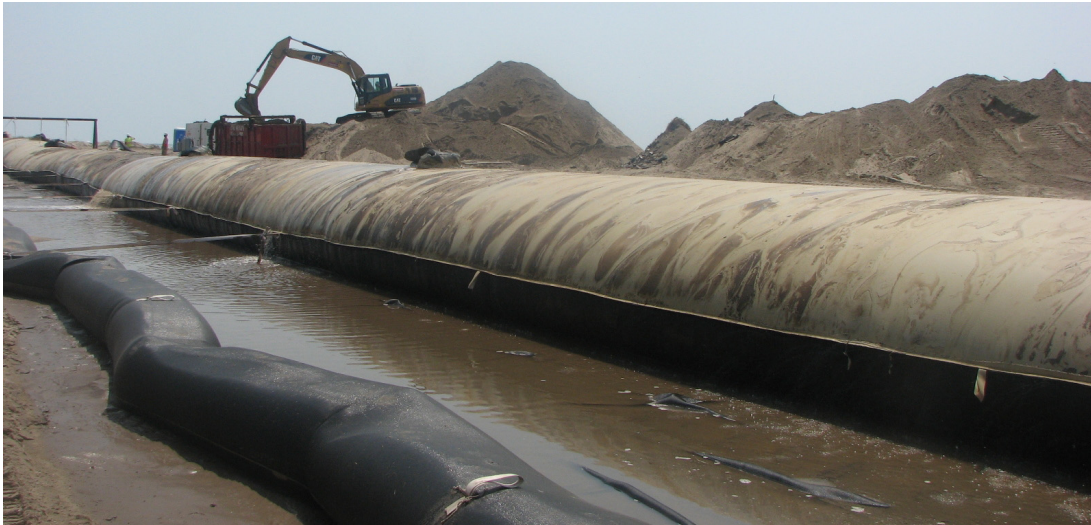
Fig. 11. Installation of geotube geotextile technology for coastal armoring [15].
