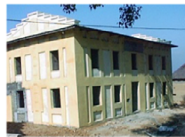
(c) After construction
