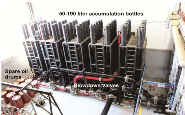
Fig. 5 – View of accumulator bank and blowdown valve
