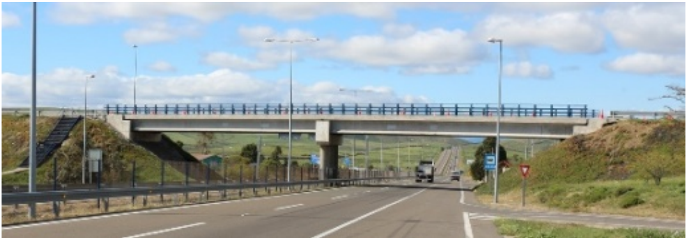
Fig. 1 – Typical Chilean overpass
