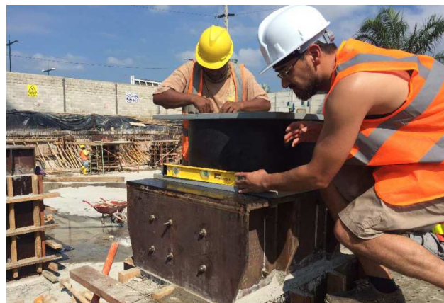
Fig. 8 – Installation of an LRB during construction
