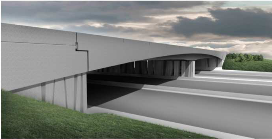
Fig. 4 – View of highway bridge at A40/A73 Interchange in Quebec, Canada
