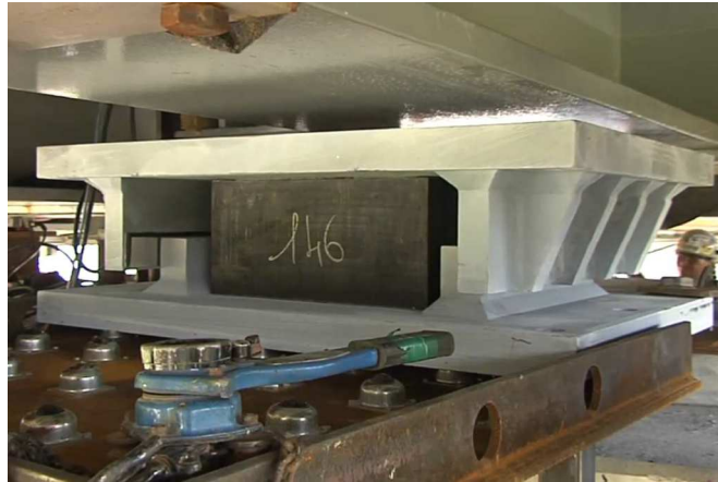
Fig. 5 – Guided lead rubber bearings installed in the bridge
