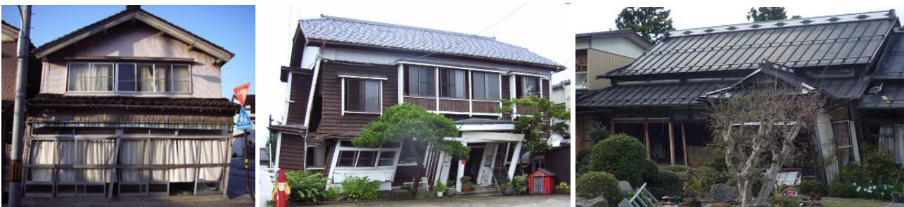
(a) 2007 Noto Peninsula quake (b) 2007 Chūetsu Offshore quake (c) 2011 Great East Japan Earthquake Photo 3 – Wood houses with large residual story deformation
