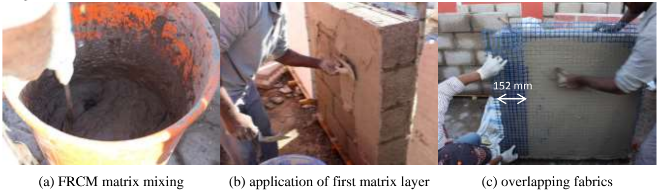
Fig. 2 – Photos of FRCM strengthening application
