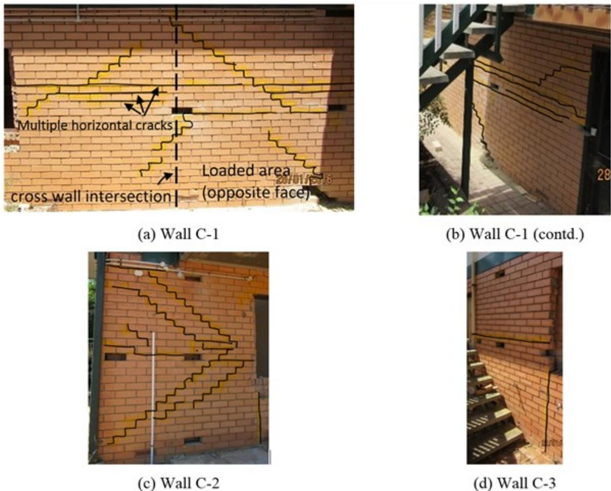
Figure 9: Crack pattern for walls in Building C
