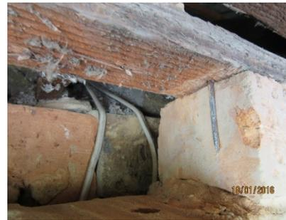
(b) Nailed connection of the timber plate to external wall leaf
