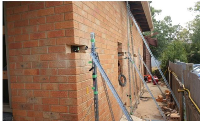
(b) Typical instrumentation (Wall A-2)
