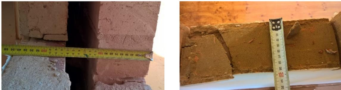
(a) Wall B-2 (typical external wall in Buildings A and B)      (b) Wall A-3 (typical internal wall in Buildings A and B)
