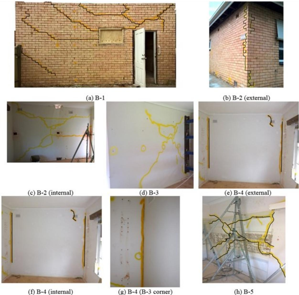
Figure 8: Crack pattern for walls in Building B
