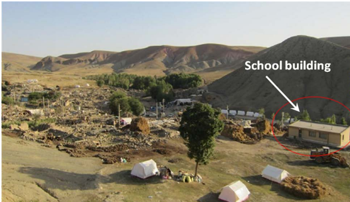
Fig.16- Example of a survived shotcreted masonry school building after Ahar earthquake of 2012
