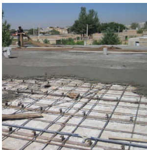
A) Lying reinforce concrete layer on top of the slab
