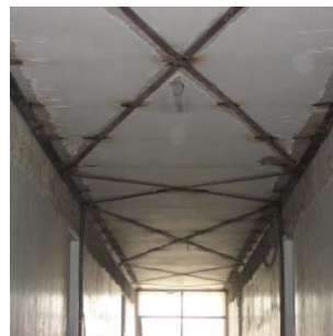
B) Diagonal steel bracing
