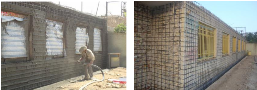
Fig. 7- Samples of retrofitted school buildings with peripheral shotcrete ( www.dres.ir )
