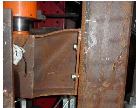
Fig.11 – The shear failure of beam
