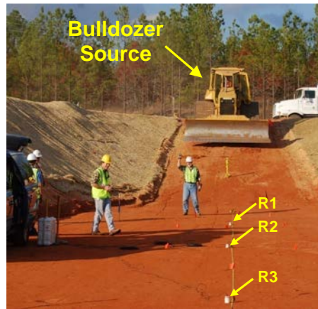
(b) SASW testing in progress at Stage 2; fill thickness \sim 3 m
