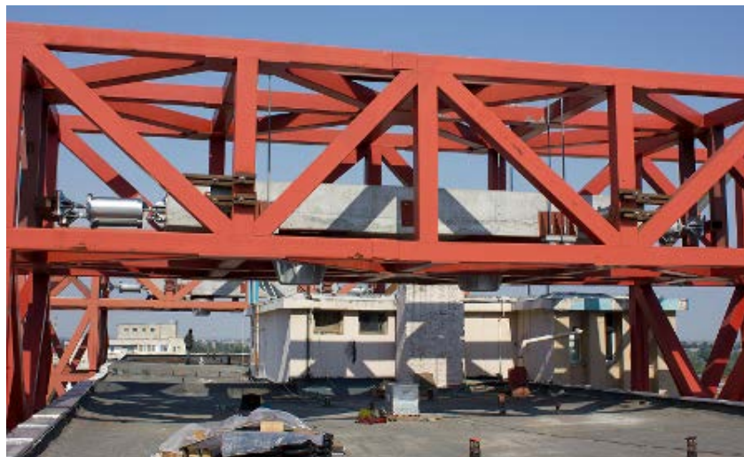
Fig. 10 – Tuned mass inside steel frame
