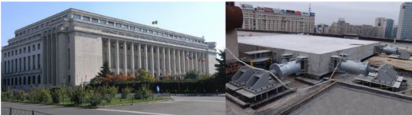
Fig. 1 – Front view of Palatul Victoria (left side) and TMCS at its roof (right side)
