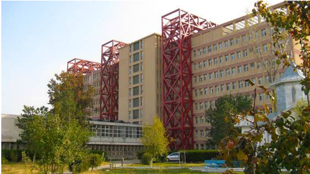
Fig. 9 – Hospital after renovation and arrangement of steel frames
