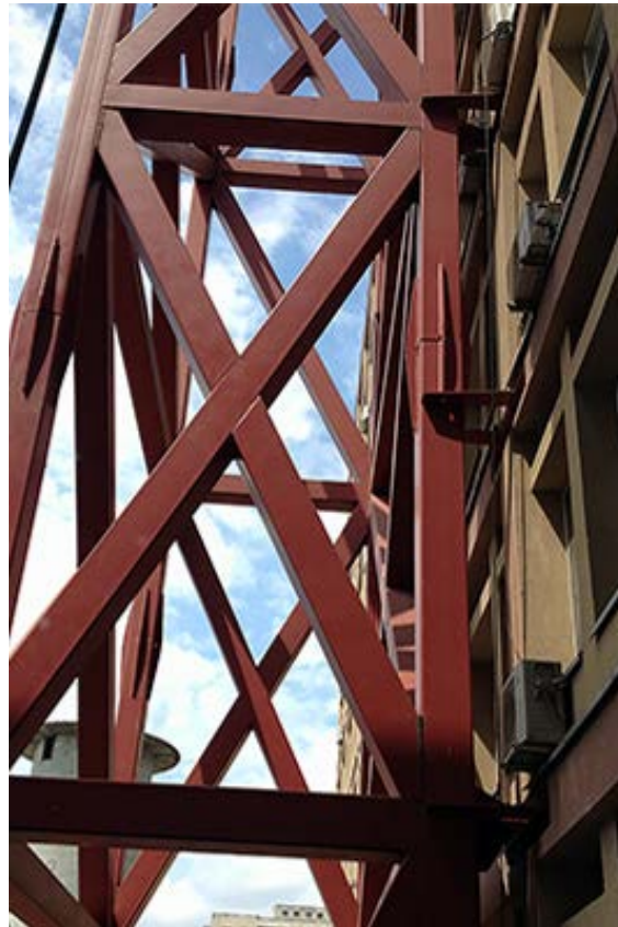
Fig. 7 – Connection between steel frame and building
