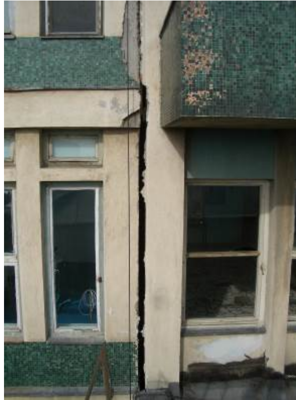
Fig. 6 – Seismic gap between two building parts
