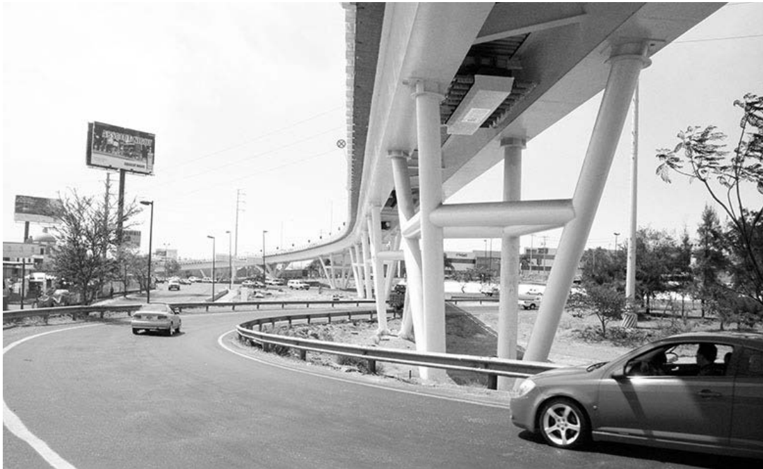
Fig. 4 – TMCS below bridge deck
