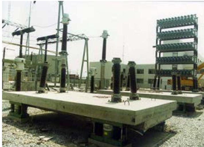
Fig. 7 – Capacitor banks on BCS
