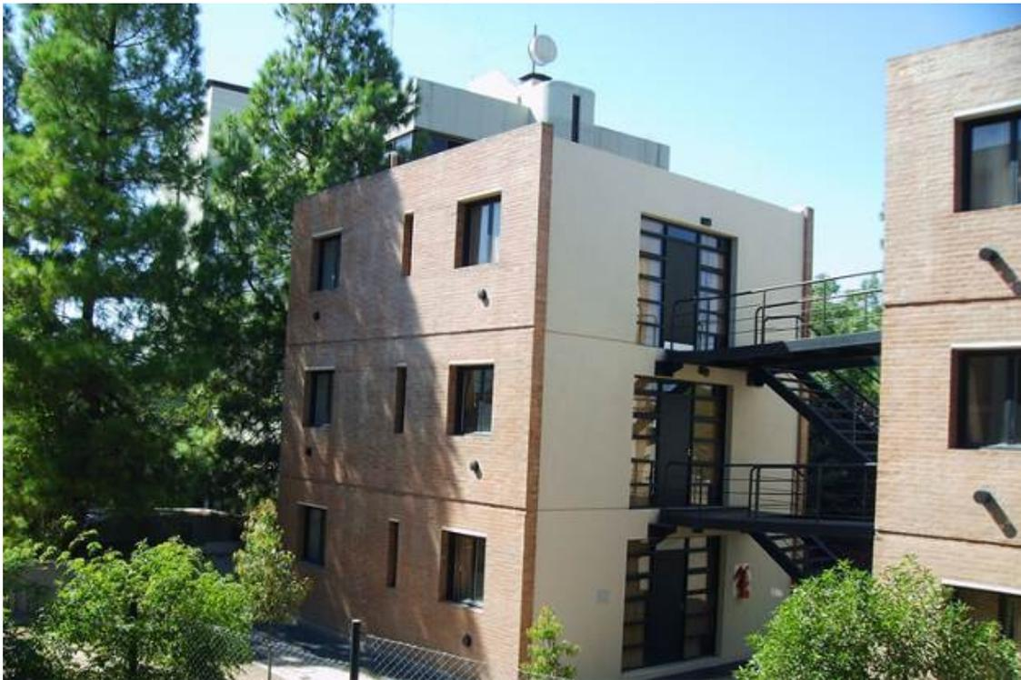
Fig. 3 – Building with rigid base (right side) and supported on a BCS (left side)
