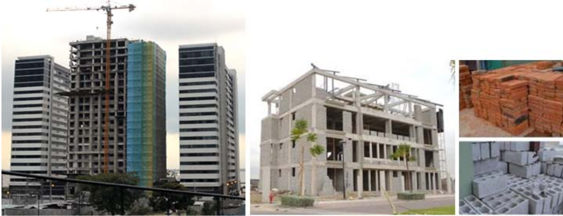
Fig. 1 – Typical RC frame buildings under construction and common masonry materials
