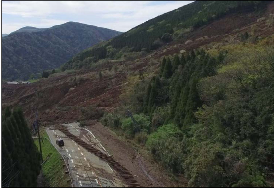
Figure 2. Railway track was dislocated by landslide.
