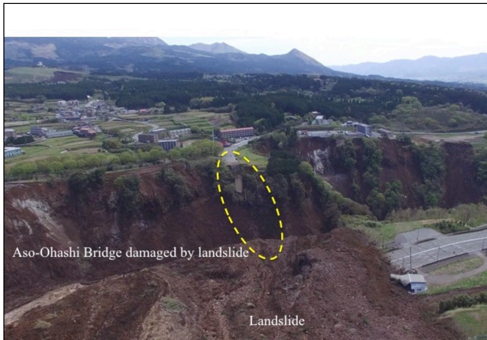
Figure 1. Aso-Ohashi Bridge was damaged by massive landslide
