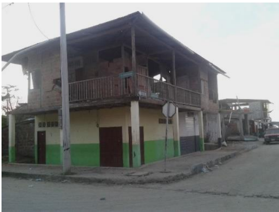
Fig. 5 – Damaged wooden structures with slender partitions made by thin clay bricks and/or concrete blocks
