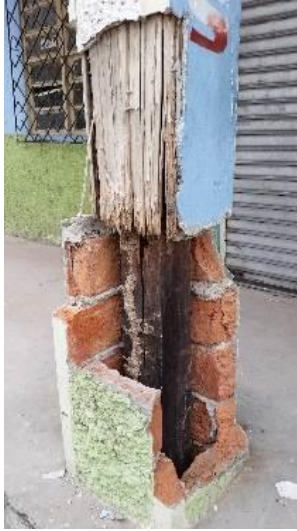
Fig. 3 – (Left) False clay brick column surrounding an existing old and deteriorated wooden column, covered by cement mortar and paint. (Right) Some non-engineered expanded constructions creating columns without continuity in all floors
