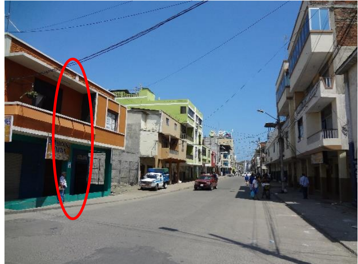
Fig. 3 – (Left) False clay brick column surrounding an existing old and deteriorated wooden column, covered by cement mortar and paint. (Right) Some non-engineered expanded constructions creating columns without continuity in all floors
