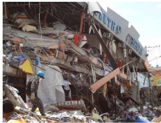
Fig. 6 – Hotel in Pedernales (left) and commercial building in Portoviejo (right). Both were expanded by the owners and converted from low rise to medium rise buildings without engineering considerations. The building at the right caused 92 fatalities (entire families) due to its collapse after the earthquake
