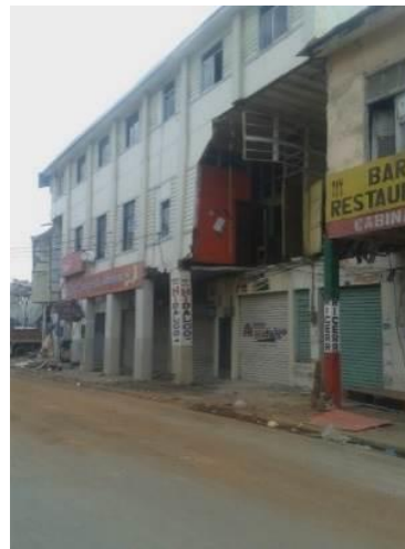
Fig. 5 – Damaged wooden structures with slender partitions made by thin clay bricks and/or concrete blocks
