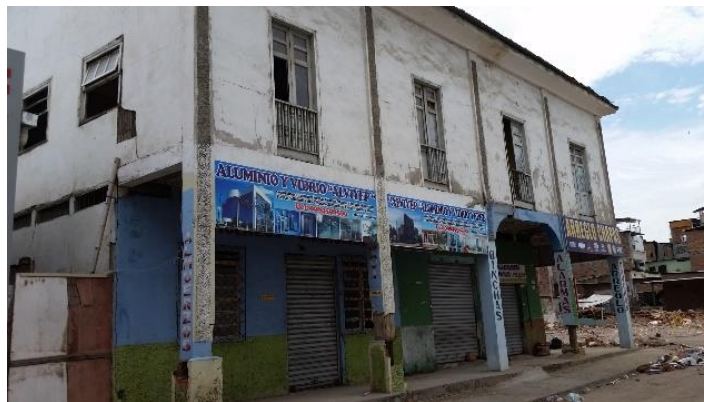
Fig. 2 – Typical wooden structures in the area, using wooden columns, beams, floor and roof system, and wooden cane, clay brick and/or concrete block units for masonry walls and partitions. External portals are common in order to permit people's circulation on streets
