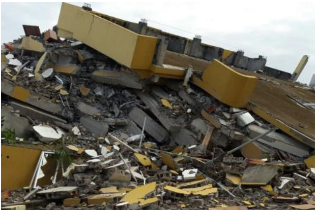
Fig. 6 – Hotel in Pedernales (left) and commercial building in Portoviejo (right). Both were expanded by the owners and converted from low rise to medium rise buildings without engineering considerations. The building at the right caused 92 fatalities (entire families) due to its collapse after the earthquake
