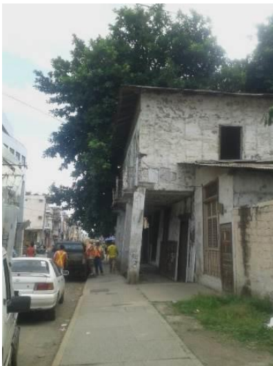
Fig. 2 – Typical wooden structures in the area, using wooden columns, beams, floor and roof system, and wooden cane, clay brick and/or concrete block units for masonry walls and partitions. External portals are common in order to permit people's circulation on streets
