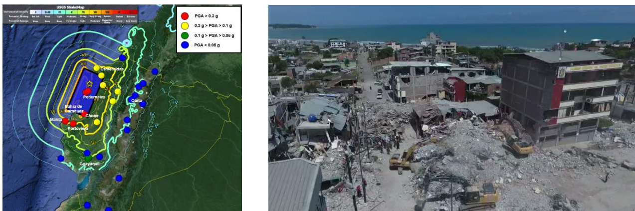
Fig. 1 – Map of the epicenter and PGA recorded of the Mw7.8 Pedernales earthquake at the north-west coast of Ecuador [1], and view of Pedernales City, where 80% of buildings were severely damaged or destroyed
