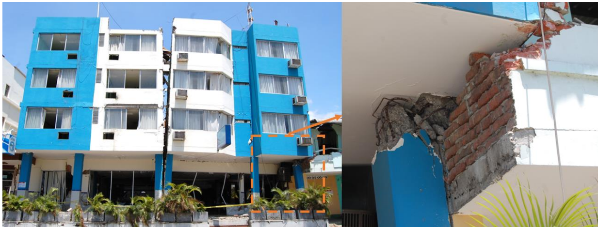
Fig.15: Pounding evidence in Hotel Las Gaviotas in Tarqui, Manta (GPS coordinates: 0^{\circ}57'6.08''S , 80^{\circ}42'48.85''W ) (Photos by GMSLLP & C. Arteta Torrents)
