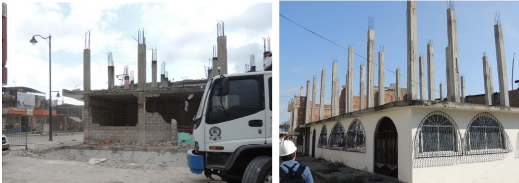
Fig. 24: Dowels sticking out from the top of the columns, presumably so a floor could be added to the building in the future a) Buildings in the coastal strip of Pedernales (GPS coordinates: 0°4'4.8"N, 80°3'23.5"W) b) Pedernales (GPS coordinates: 0°4'4.8"N, 80°3'23.5"W) and Tarqui, Manta (GPS coordinates: 0°57'9.04"S, 80°42'41.54"W). (Photos by GMSLLP)
