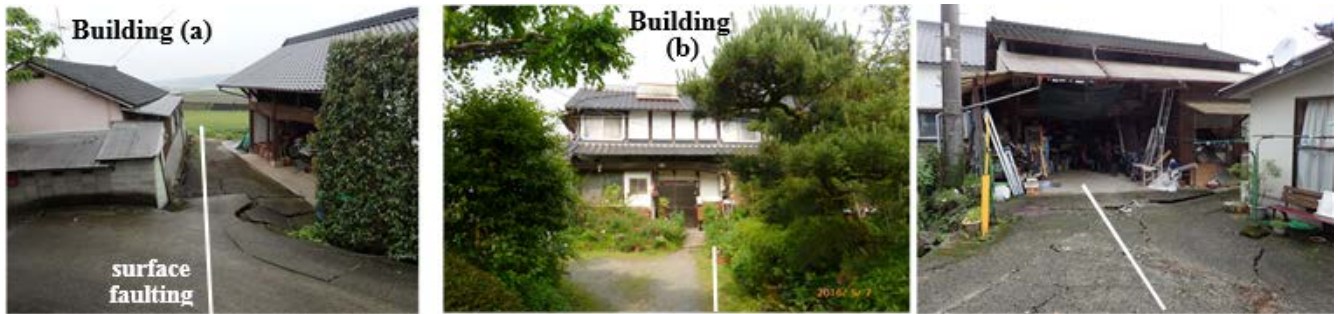
(a) An old wooden house (left) on the surface fault (Damage grade 3) (b) A very old wooden house on the surface fault of the front (left: Damage grade 3), and the back (right: a very old warehouse of damage grade 1)
